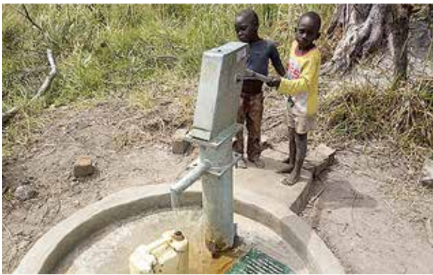
Photo Courtesy of Aid Africa The Aid Africa organization digs and repairs wells for villages in Uganda, Africa, providing clean water that is easily accessible to residents, eliminating the need to fetch water from great distances.
