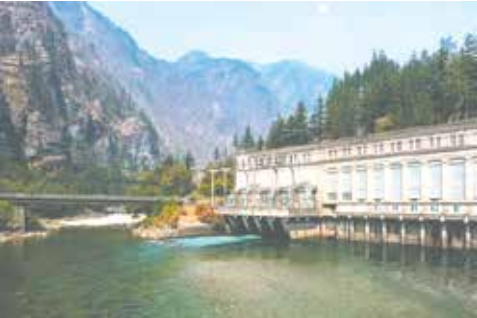
The Gorge Dam Power House on the upper Skagit River.
